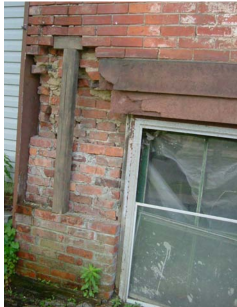
Missing bricks have left the northeast wall very thin and action should be taken immediately to reconstruct the wall.
