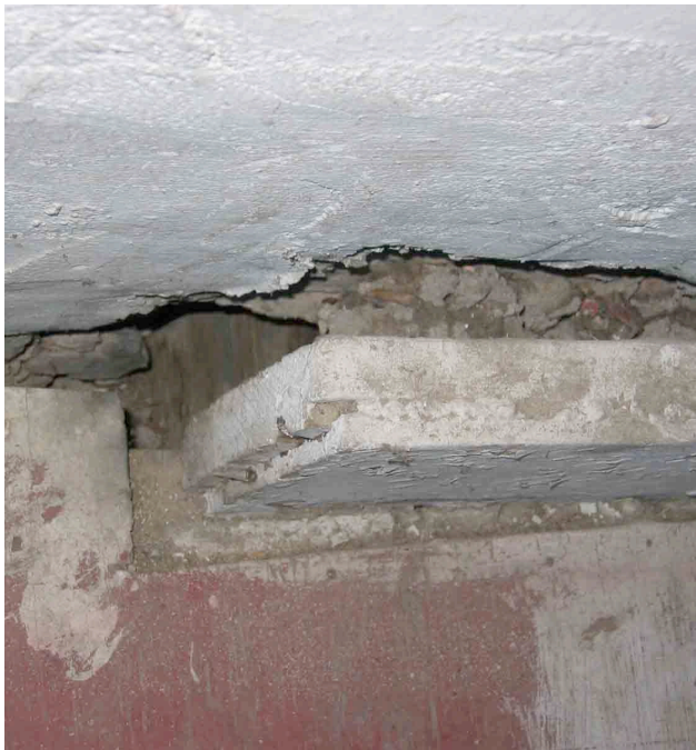
Photograph No. 15. View of another landing of the main staircase where the header and the stair have moved away from the interior face of the exterior wall.
