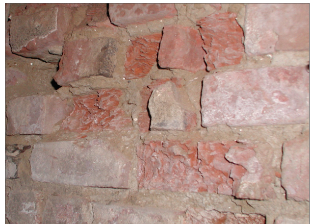
Figure 54: Repeat freeze and thaw cycles have left the bricks in the basement walls brittle and friable.
