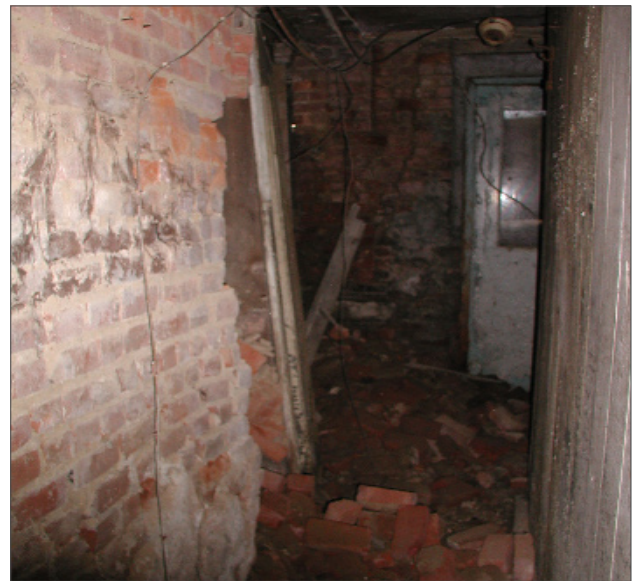
Figure 53: The south end of the brick stiffening wall between the basement hall (B03) and the former kitchen (B02) has suffered partial collapse.
