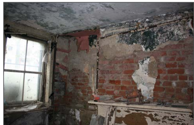
Figure 55: Most of the finishes in the basement are deteriorated from water infiltration. Plaster from the walls and chimney breast in the northeast corner of Room B01 have delaminated from the brick walls.
