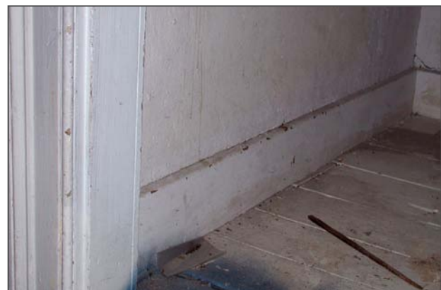
Figure 109: Room 204 is the only room in the entire house that retains original baseboards. The baseboard is a plain board with a beveled top edge.
