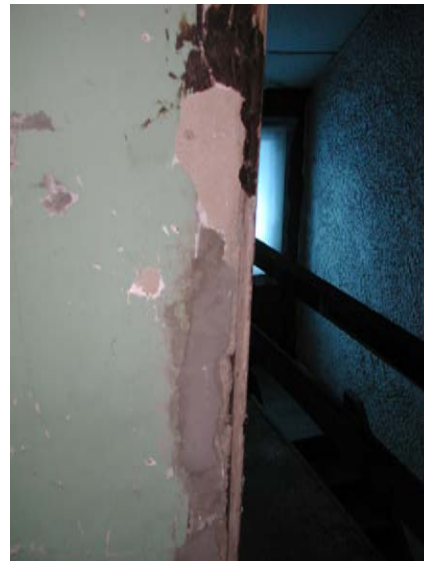
Damage to the outside corner in Room 304 exposed an original wood corner bead.
