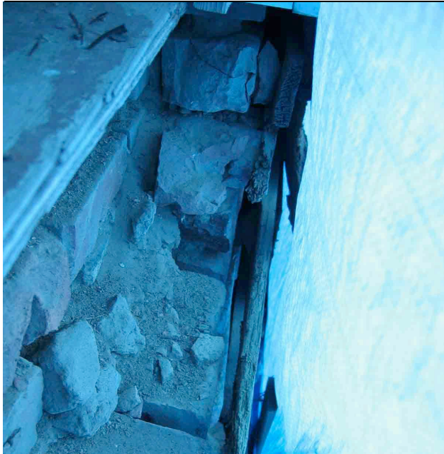
Photograph No. 13. View of the exterior brick below a second floor window sill (on the south elevation).
