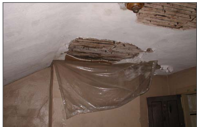
Figure 118: Damage to the plaster ceiling along the east wall in Room 301 was likely caused by water entering through failed chimney flashings.
