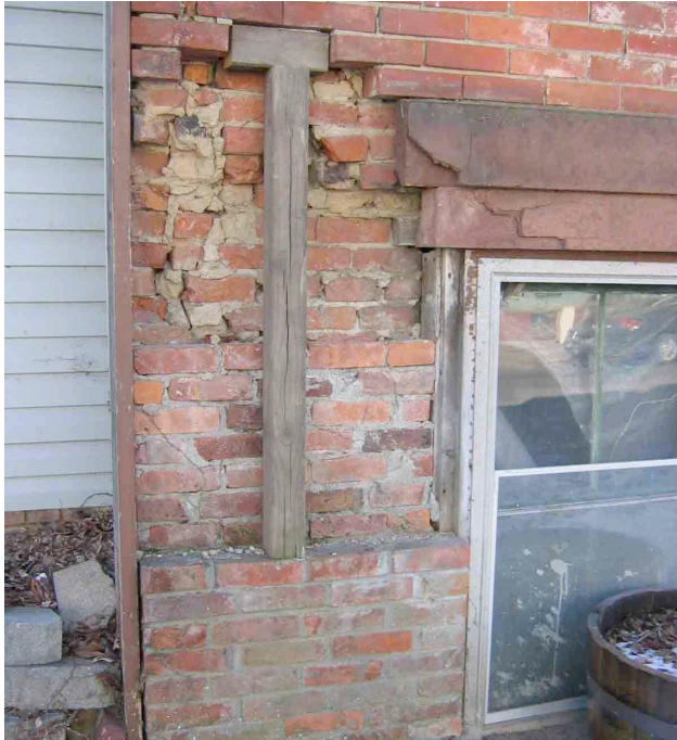
Photograph No. 17. View of localized failure of exterior wythes of brick masonry at the NE corner of the building.
