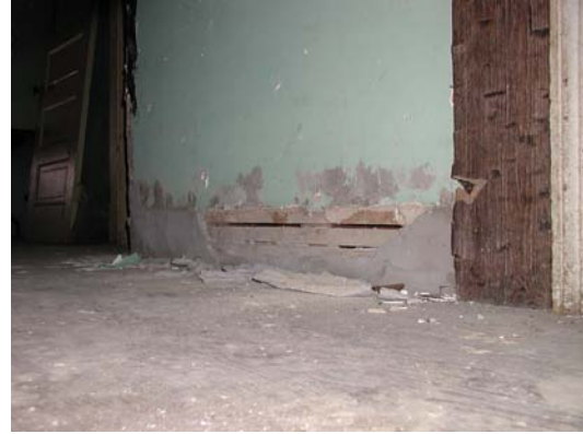
In Room 304, the baseboards were removed and the exposed space patched with cement.
