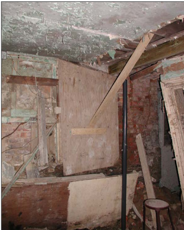
Figure 52: All of the brickwork at the south end of the stiffening partition between B02 and B03 has collapsed. Temporary posts and beam support the first floor.
