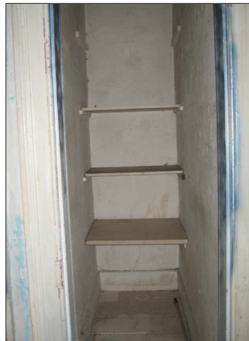
Figure 108: View of the room looking west.
