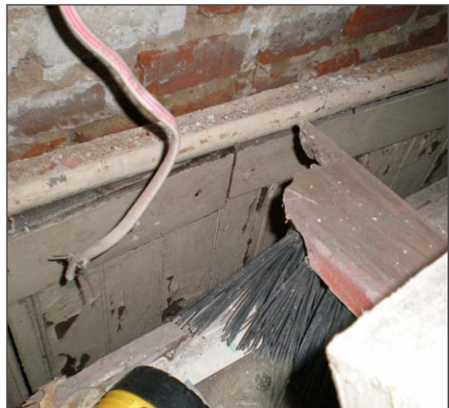
Figure 61: Intact wainscoting and chair rail on the south wall in Room B01.
