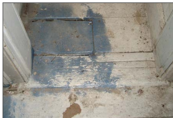
Figure 110: The east end of the floor has been cut, likely to facilitate access to the gas pipes serving the chandelier in Room 103 below.
