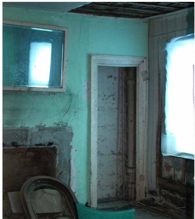
Room 202 has a shallow closet on either side of the fireplace opening. The mantelpiece was removed at an unknown date and the wall repaired with portland cement.
