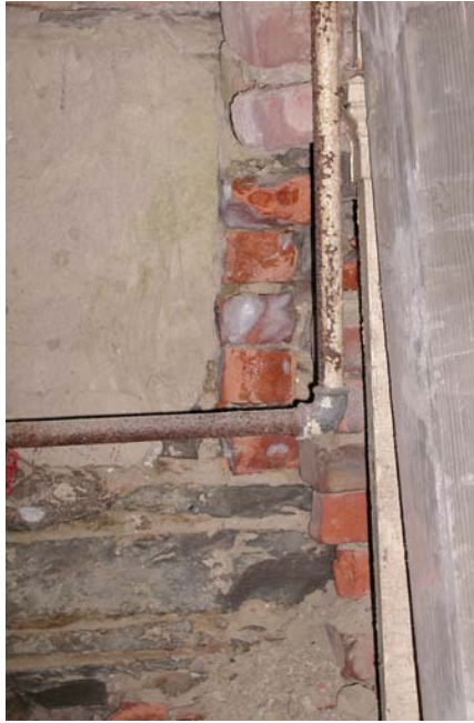
This iron pipe in Room B01 was most likely a gas pipe.
