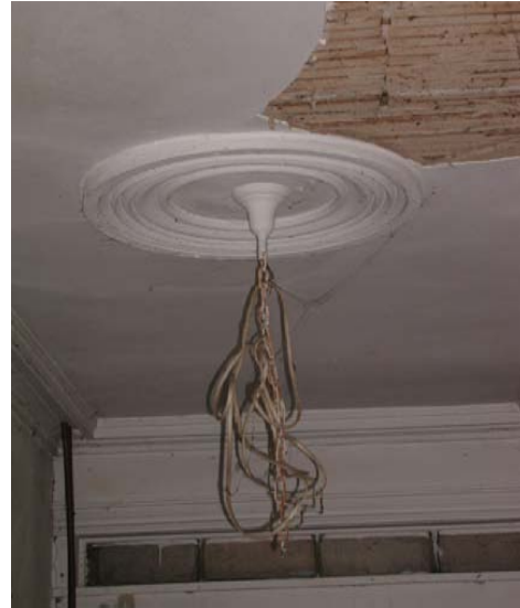
Once the Stabilization work is complete, attention can be paid to interior details such as moldings and light fixtures.
