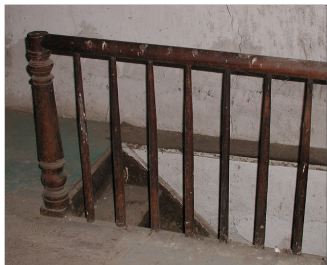
Figure 85: The stair to the cellar retains most of its original ballustrade. The cap on the newel post is missing.
