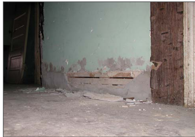
Figure 124: In Room 304, the baseboards were removed and the exposed space parged with cement.
