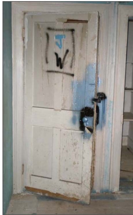
Figure 96: A four-paneled door hanging in 201 with possible original hardware, one of the few that remain.
