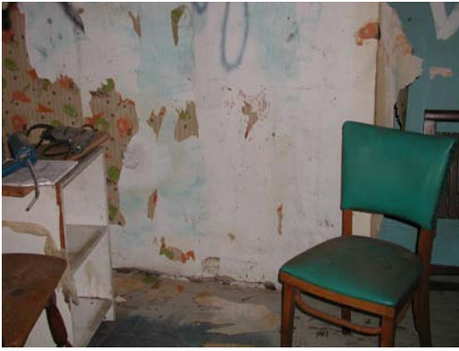
The chimney breast in Room 201 should be carefully studied.
