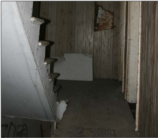
Figure 106: View of hallway and staircase on the second floor (Room 203)
