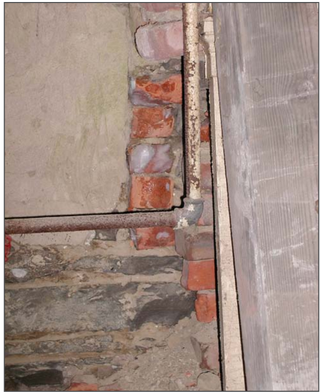
Figure 134: This iron pipe in Room B01 was likely a gas pipe.
