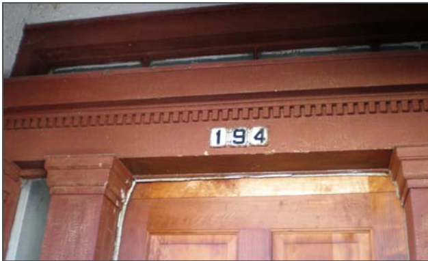
Figure 88: Detail of wooden frontispiece with dentil cornice.
