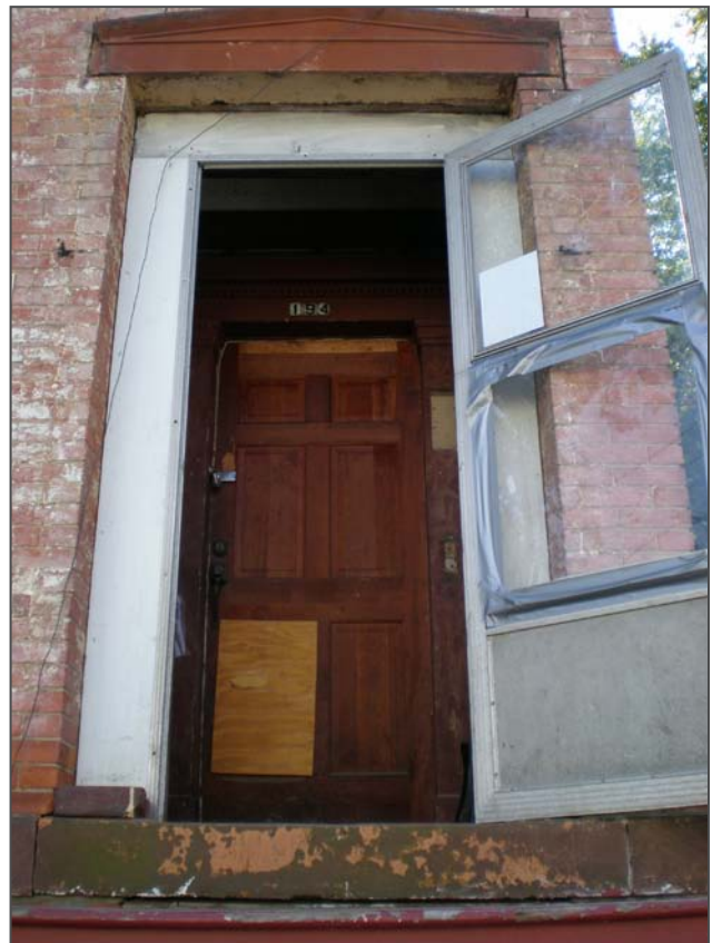
Figure 87: North entrance with screen door and sandstone sill, looking at frontispiece.
