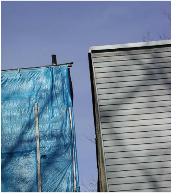
The masonry at the gable end on the east façade is visibly bulging.
