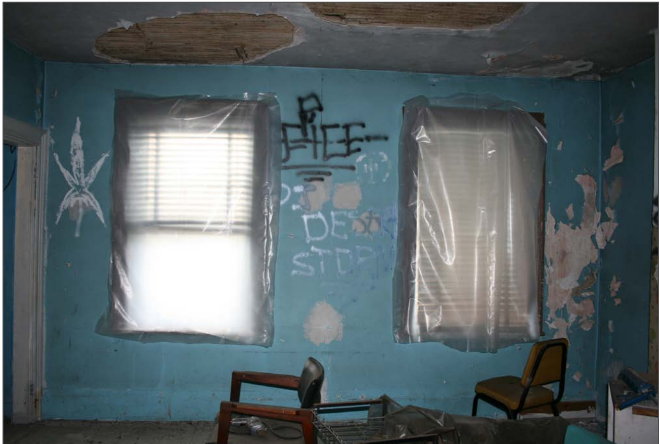
Figure 97: Two windows on the north facade illuminate this room.
