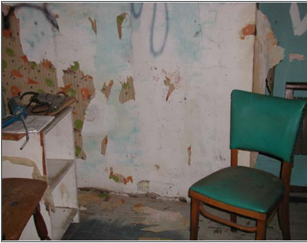
Figure 92: The chimney breast in Room 201 is currently covered in GWB .
