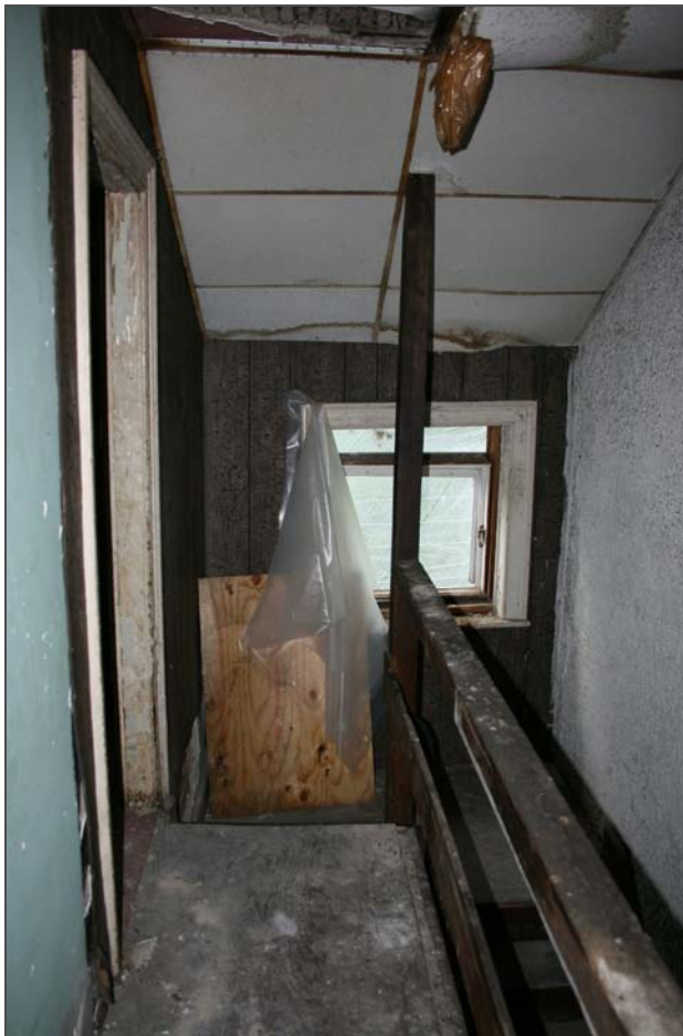
Figure 125: View looking south into the north-south corridor of Room 304.
