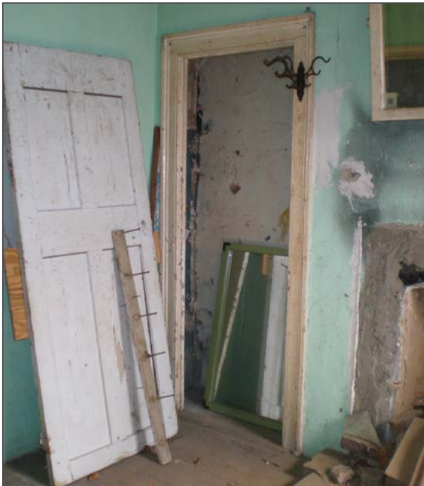
Figure 98: An original door with original hinges was found in Room 202.
