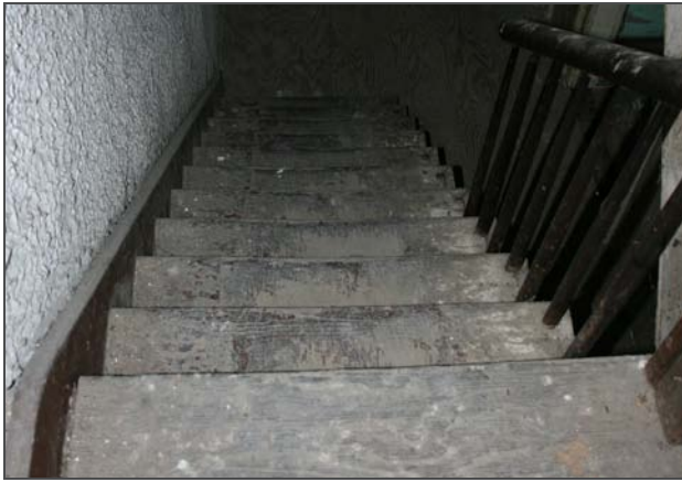
Figure 105: Stairs to the third floor with remaining railing and balusters.
