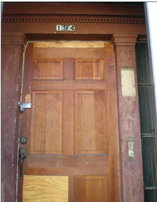
Figure 89: Contemporary door replacement on frontispiece on the south wall of Room 104.
