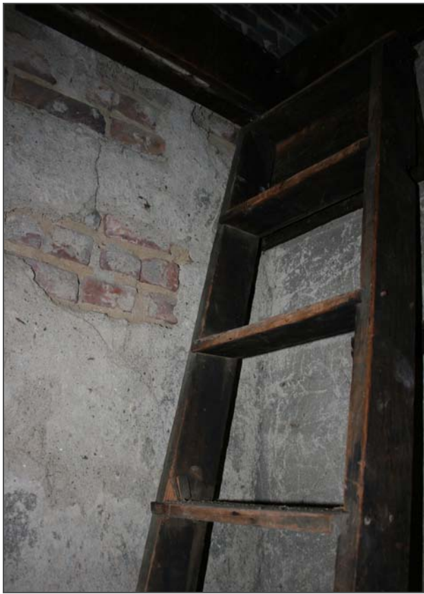
Figure 130: The ladder in Room 305 that accesses the attic.
