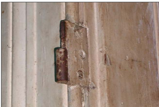
Figure 102: This lift-off hinge was found in Room 202. It was the only example of this type of hinge found in the building.
