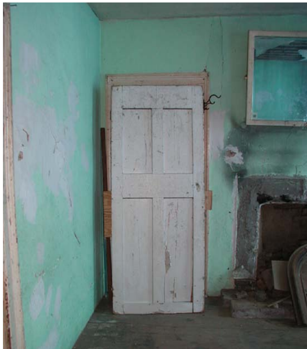
An original door with original hinges was found in Room 202.
