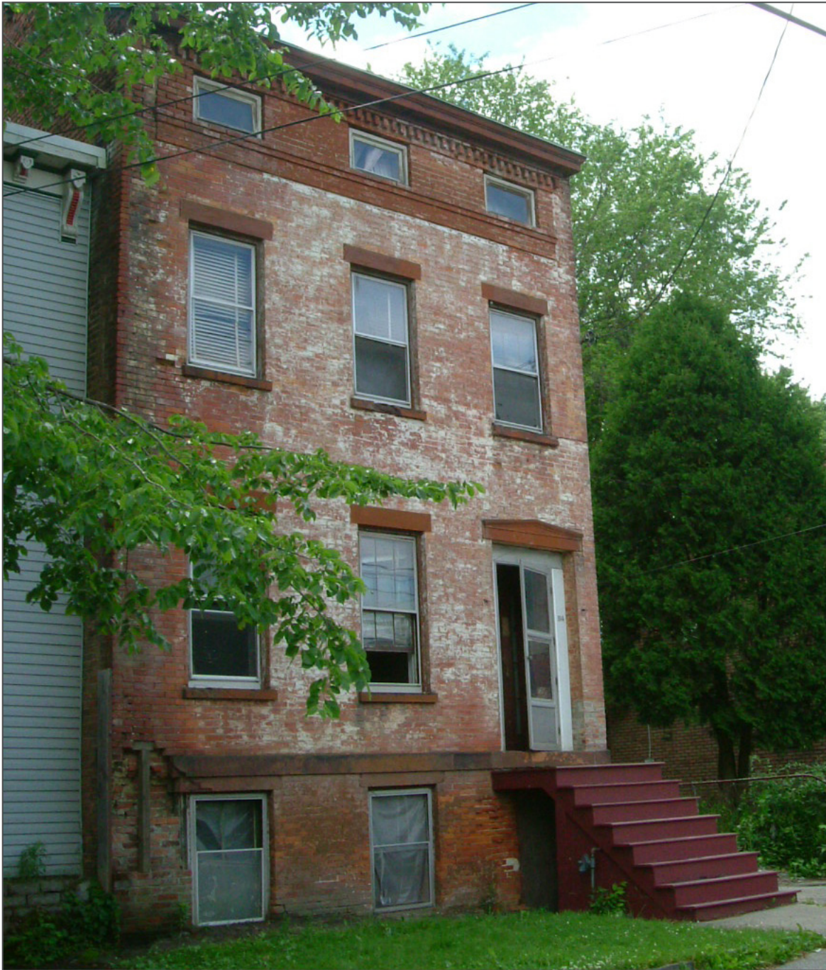
Figure 1: Front (north) facade of the Myers Residence.
