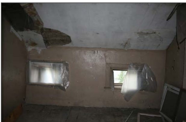
Figure 117: Two north-facing windows and sloping ceiling.
