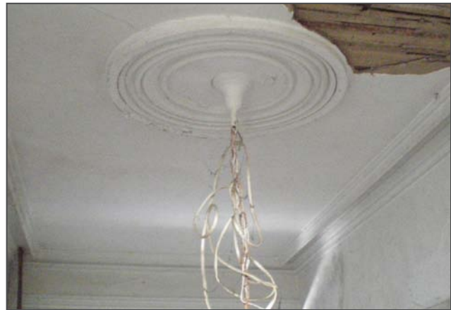
Figure 84: Central ceiling medallion with wiring and chain remaining from previous fixture.
