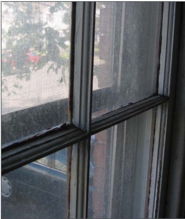
Figure 75: Detail of muntin profile on East window in Room 101, likely original.
