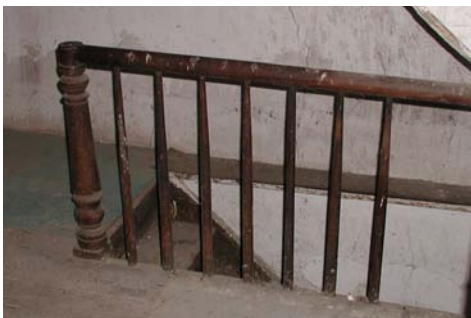
The stair to the Cellar retains most of its original ballustrade.
