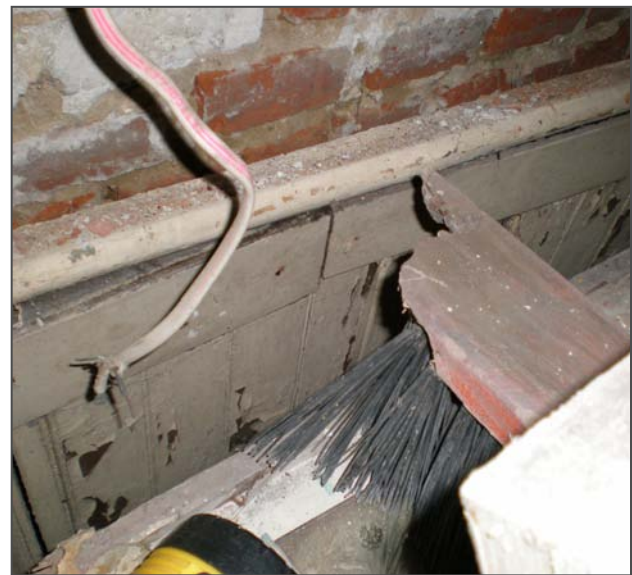
Figure 61: Intact wainscoting and chair rail on the south wall in Room B01.
