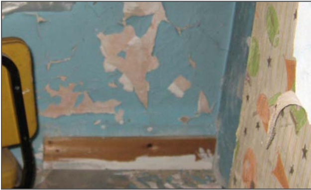
Figure 93: A small area of “modern” baseboard in the northwest corner.
