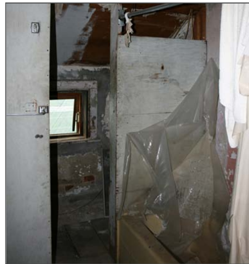
Figure 119: View looking south with tub and window in Room 302.
