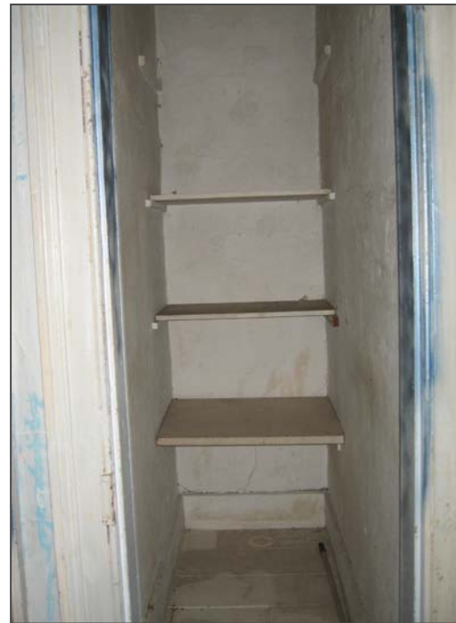
Figure 108: View of the room looking west.
