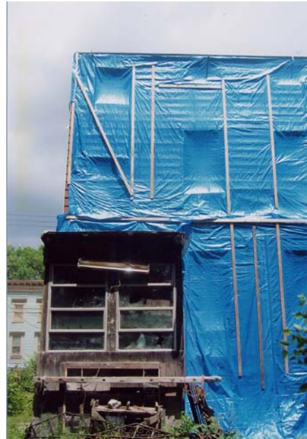
The south façade is presently covered in tarps to stop ongoing water infiltration. The rear porch, a later addition, is probably not salvageable.
